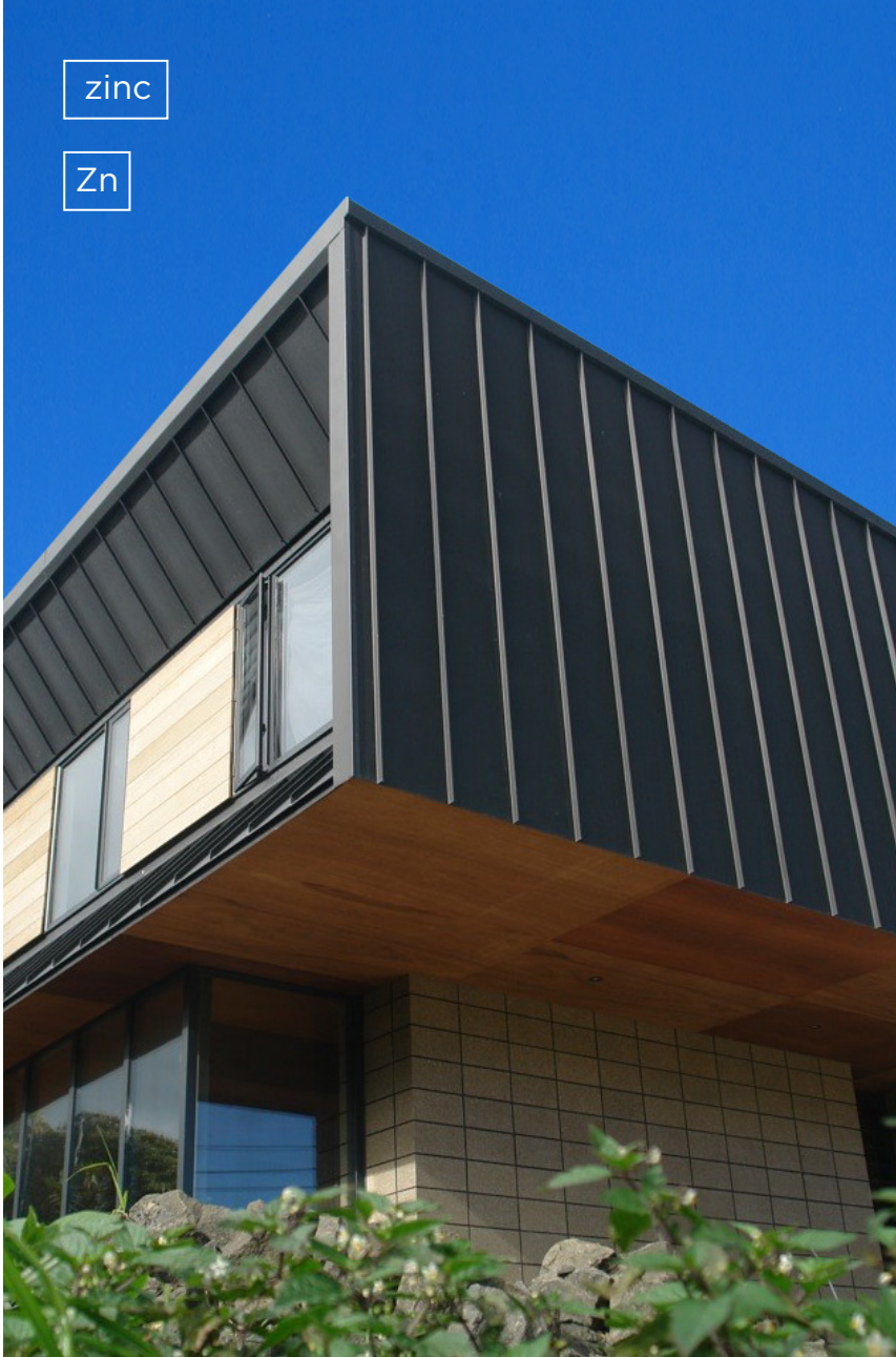
Smart Tray Metal Cladding Standing Seam 0.7mm Zinc Cladding.
