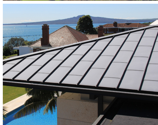
Smart Tray™ Custom Panel 0.9mm Aluminium Roof on the ASB Head Office in the Wynyard Quarter.
