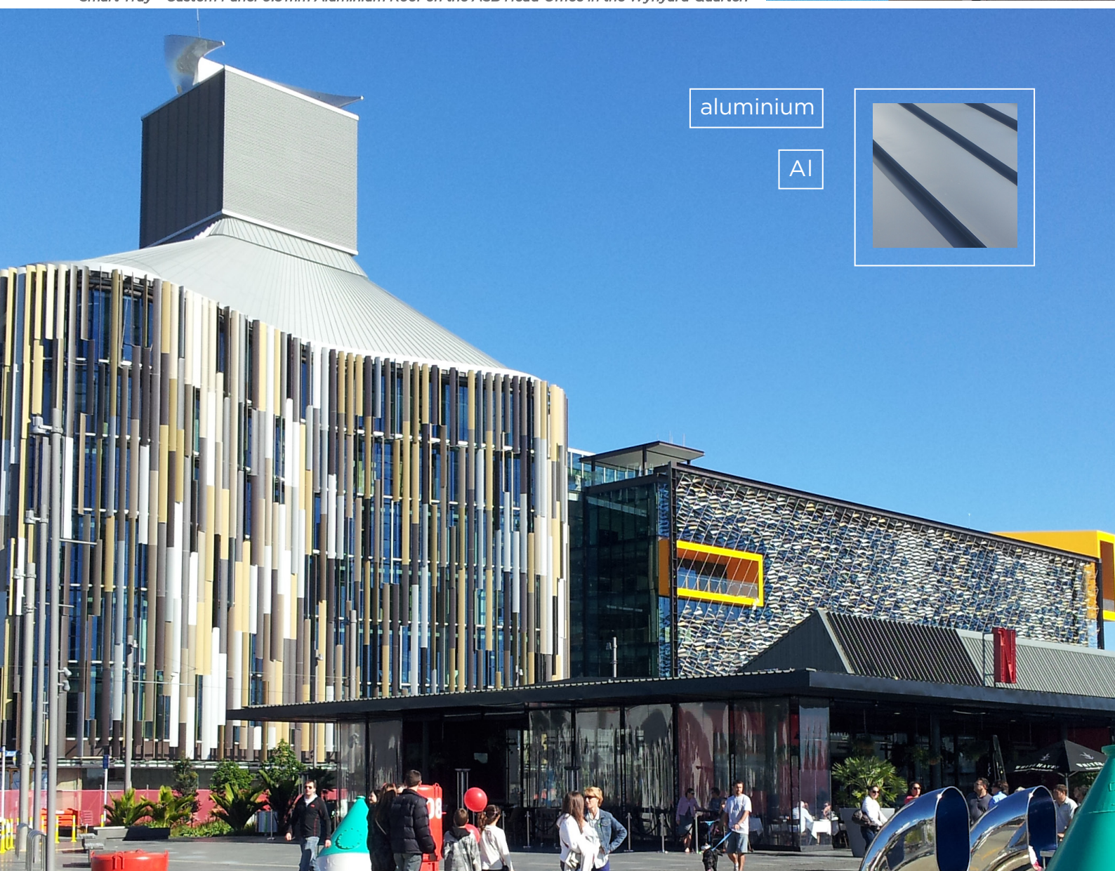
Smart Tray™ Custom Panel 0.9mm Aluminium Roof on the ASB Head Office in the Wynyard Quarter.
